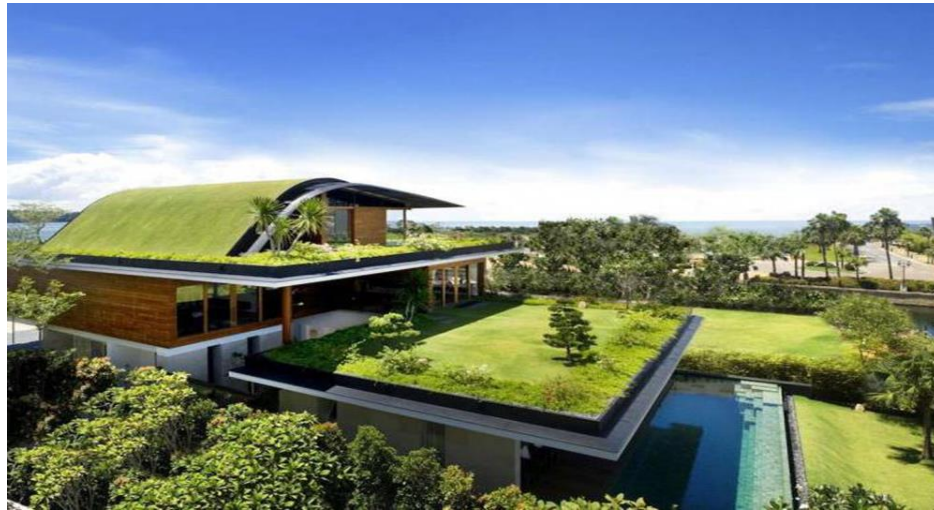
Figure 3- Eco-roofs designed for walking, relaxing or placing greenhouses
