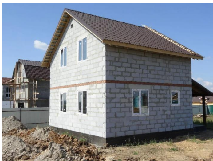
Figure 1 - The construction of gas silicate blocks
