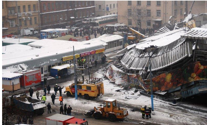
Fig. 3. The Basmanny Market building in Moscow
